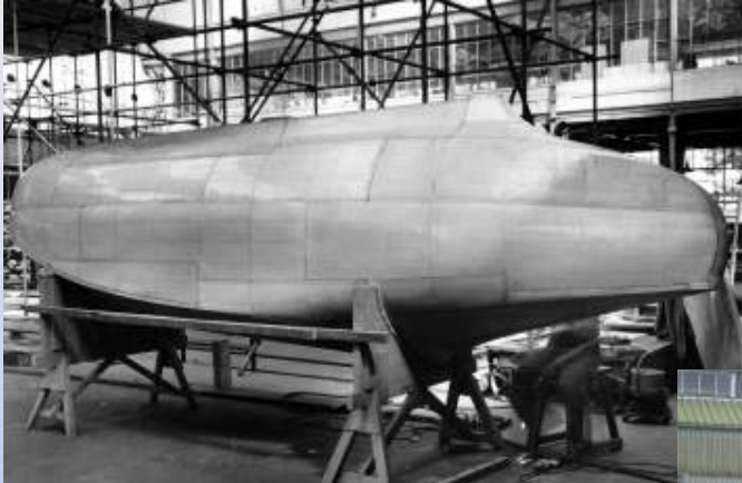
Princess float under construction c1951
